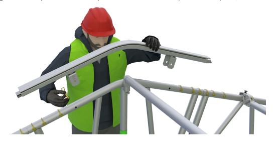
Slide the relevant DeepFlow $^{\text{TM}}$  track length up the slope of the beam line with the spigot pointing downslope and with the label pointing upslope, making sure the tracking engages with the button nuts attached to the brace claws.
